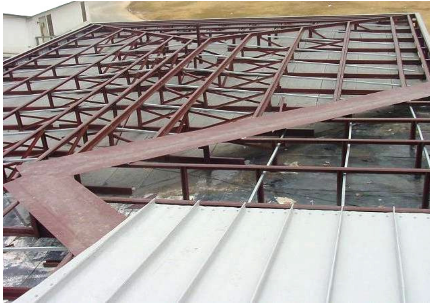
Typical low-slope application over nearly flat roof
